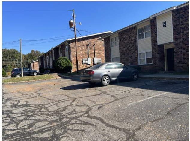
Subject parking area
