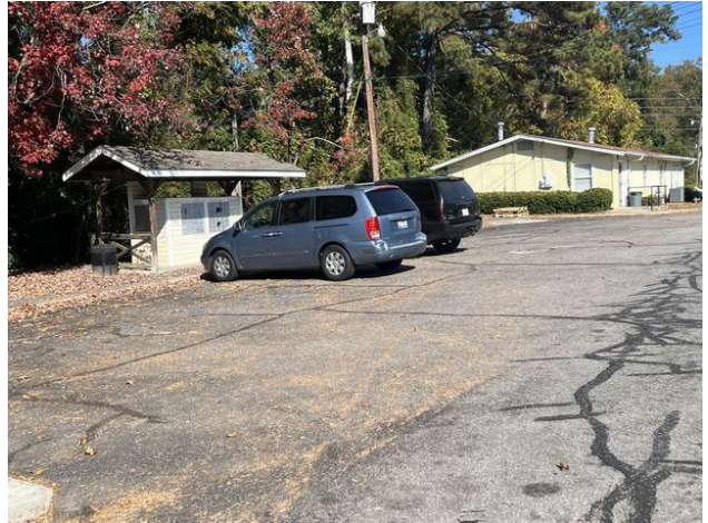
Mail area & community building/leasing office
