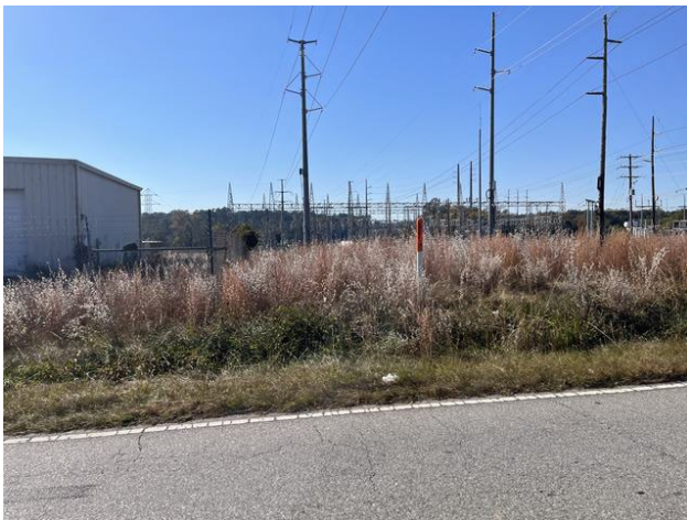
Electrical substation north of Subject
